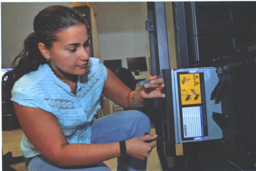
FAU student Vanessa L. Diaz inspects a component of the IBM Blade Center, part of the university's supercomputer cluster.
